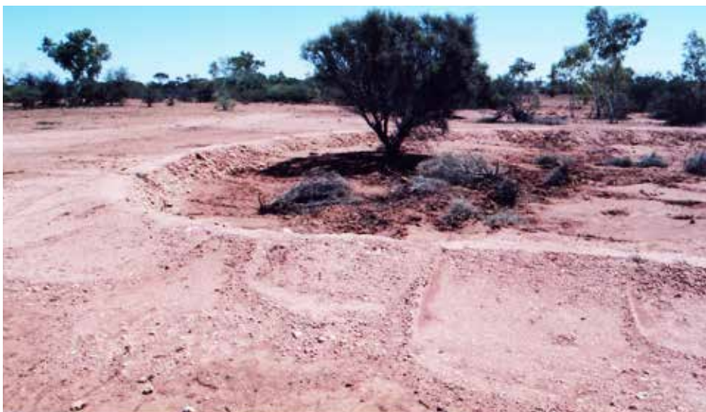
Figure 41: A six photo sequence of stabilising shallow gully heads using calcrete rubble bunds.
